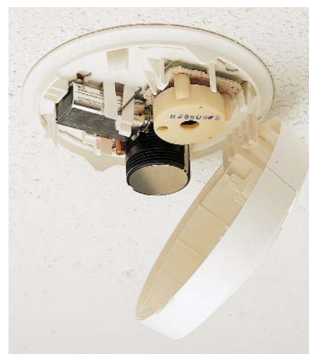
Figure 7-12 In a smoke alarm, a small alpha-emitting isotope detects smoke particles in the air.
