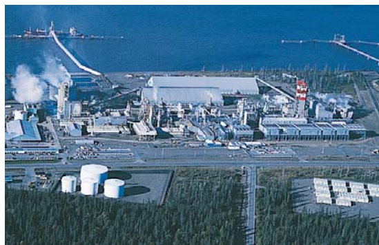
Figure 5-24 Ammonia, which is manufactured in plants such as this, is used to make ammonium perchlorate—one of the space shuttle's fuels.
